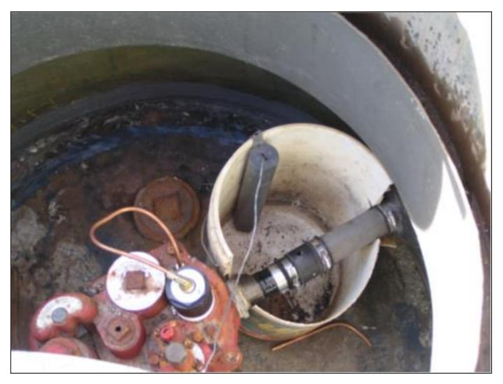
While the sensor is upright, it's not in the lowest part of the containment sump and a jerry-rigged bucket is not the correct way to fix a leak.
