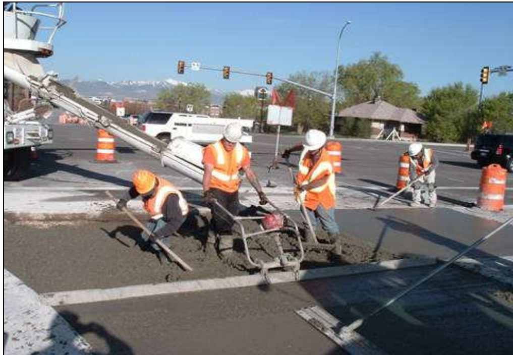
Pouring new concrete road panel on Sego Lily Dr at State Street
