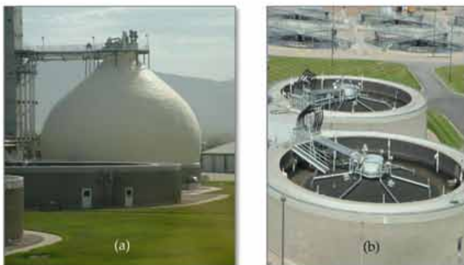
Figure 1 - Anaerobic Digestion Systems at the Central Valley WWTP: (a) Egg-Shaped Digester; (b) Conventional Floating Roof Digesters
