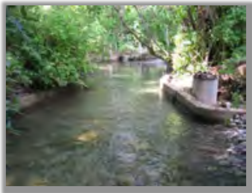
Submerged Parshall Flume (Smithfield, UT)
