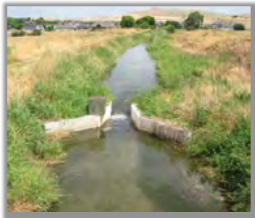
Parshall Flume (Smithfield, UT)
