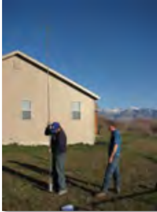
Deep trench installation, Clarkston, November 2008
