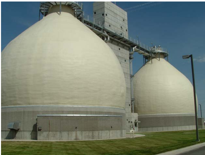
Figure 1. Anaerobic Digesters - Central Valley Wastewater Treatment Plant – Salt Lake City, Utah
