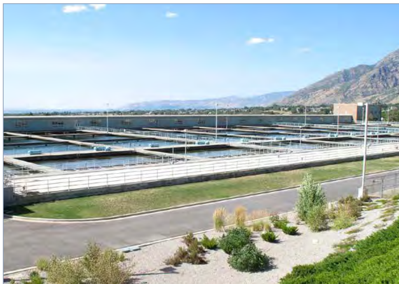
Figure 1: Little Cottonwood treatment plant ponds.
