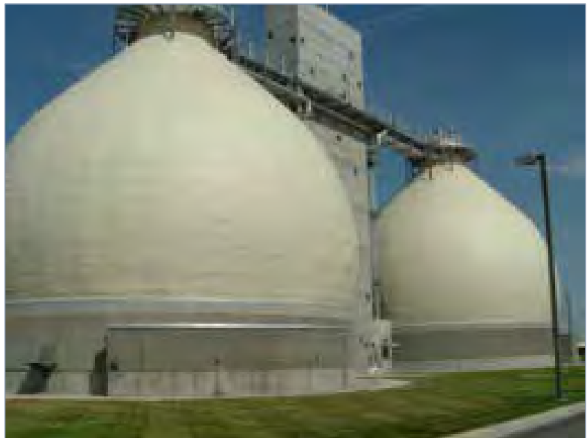
Figure 1: Anaerobic Digester System at Central Valley Water Reclamation Plant (Salt Lake City, Utah).
