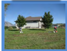
Deep trench system installation, Wellsville, November 2008.
