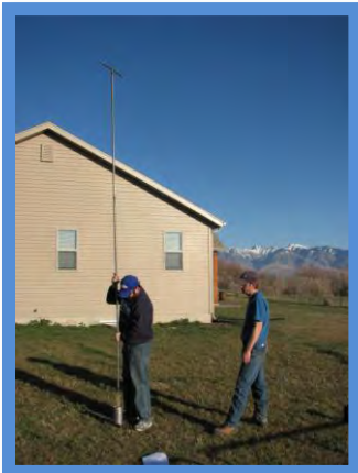
Deep trench installation, Clarkston, November 2008.
