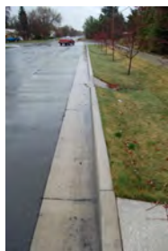
Figure 1: Stormwater BMP site, 300 E Logan.
