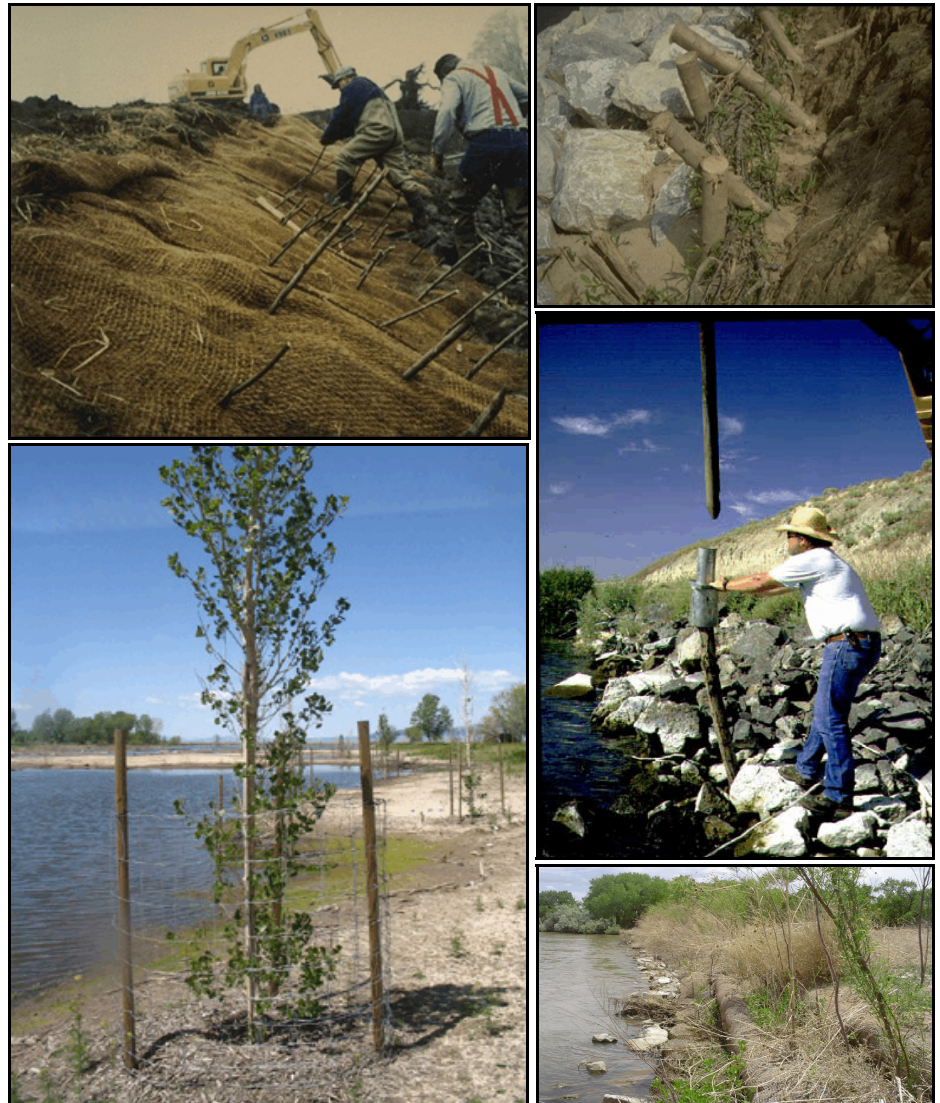
Figure 4.4. Photographs of revegetation and biotechnical slope-stabilization techniques. (Top left: erosion-control blanket and live stakes [image from FISRWG 1998]. Top right: live pole plantings [image from FISRWG 1998]. Bottom left: containerized cottonwood ( Populus sp.) planting protected from herbivory with wire mesh cage. Middle right: installation of live plant posts to create vegetated rock revetment [image from NRCS 2007]. Bottom right: vegetated soil lifts with live plant stakes and rock toe protection.)
