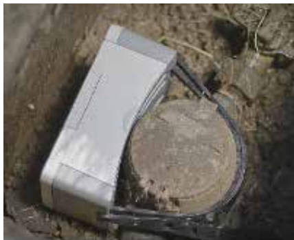
Figure 1: Flume, Inc. Smart Home Water Monitoring device (grey) strapped around a water meter.
