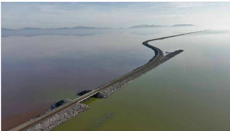
Figure 1: The Great Salt Lake's West Crack Breach
