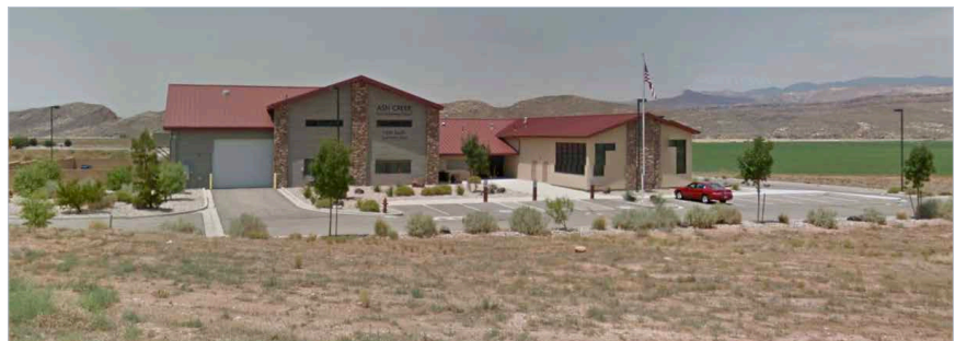
Figure 1: The new demonstration site will be located at the Ash Creek Special Service District in Hurricane, Utah.
