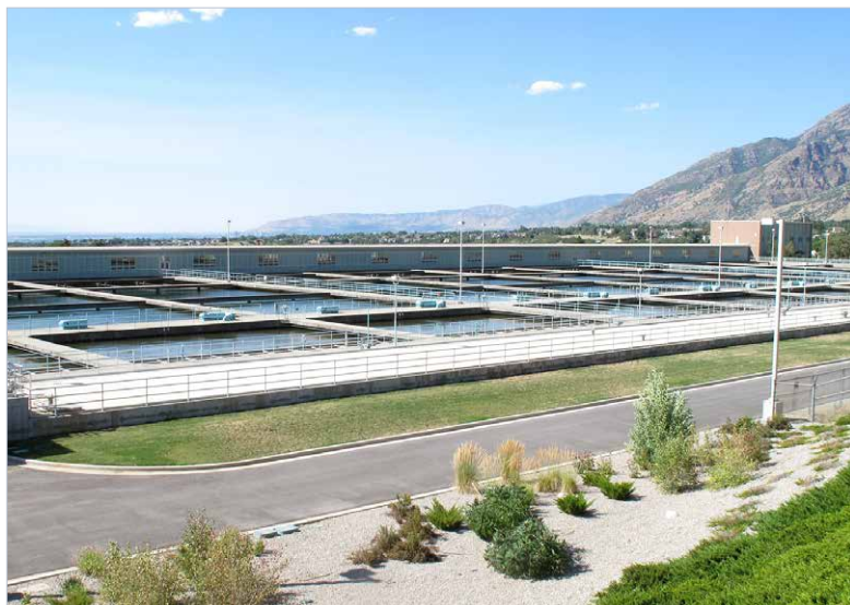
Figure 1: Little Cottonwood treatment plant ponds.
