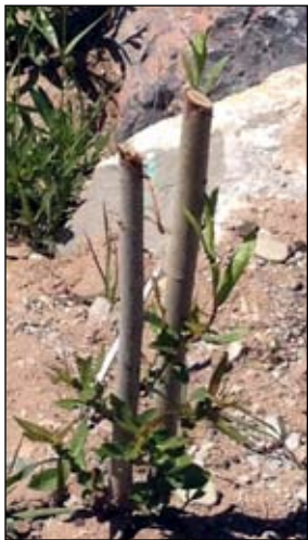
Cuttings from dormant riparian shrubs are planted deep enough in streambank soils to reach the dry season water table. These "live stakes" are used in a variety of bioengineering techniques. Stem nodes underground will take root; nodes above ground will leaf out.
