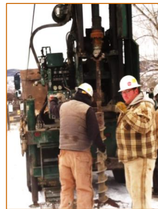
Figure 2. Drilling for water table aquifer cores
